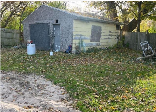
Exterior Storage Shed
